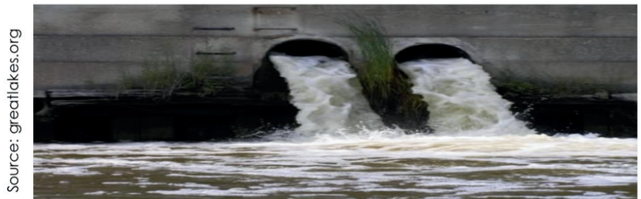
Combined Sewer Overflows (CSO), in the event of extreme rainfall, can overflow, sending raw sewage to a river or lake.
