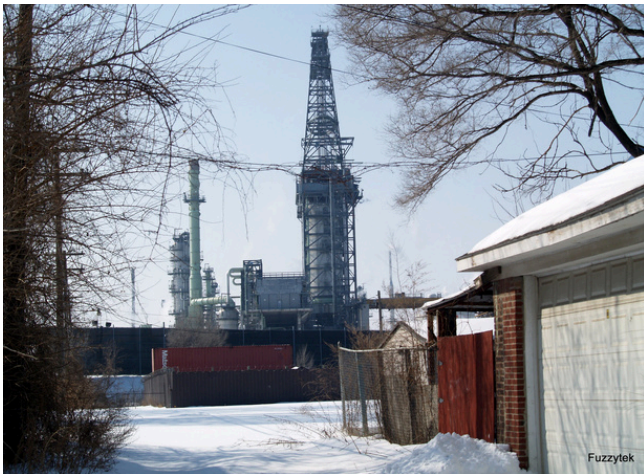
Marathon's Detroit Refinery in Oakwood Heights. Via Flickr, Creator: Stephen Boyle
